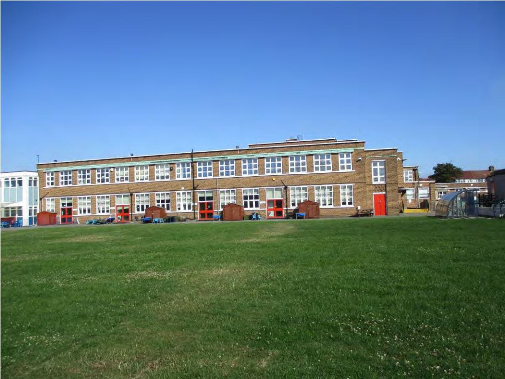
Rear elevation of main building
